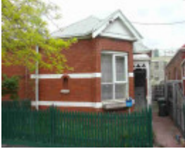
fitzroy north scotchmer street fitzroy north scotchmer street 8
