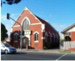
Burnley Uniting (former Presbyterian) Church
