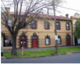
fitzroy north queens parade fitzroy north queens parade 436 unit 1
