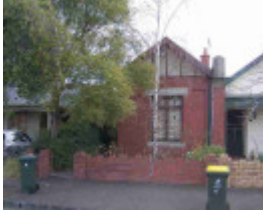
fitzroy north white street fitzroy north white street 11
