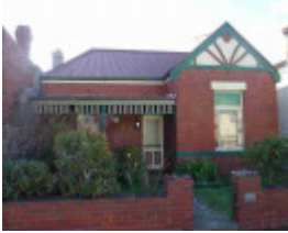
fitzroy north woodside street fitzroy north woodside street 33
