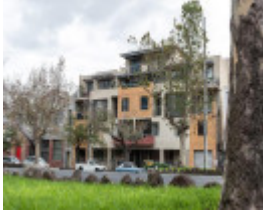
Millennium apartments facade 140 Queens Road Fitzroy North
