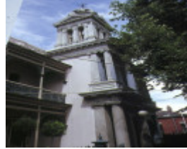
1 finn barr cecil street south melbourne tower view feb1992
