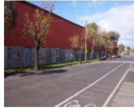
Former Coal Shed for Inner Circle Railway (Napier Street)
