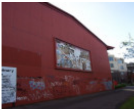
Former Coal Shed for Inner Circle Railway (Queens Parade)
