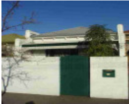
fitzroy north woodside street fitzroy north woodside street 22
