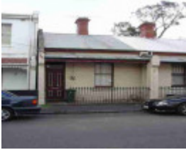
fitzroy argyle street fitzroy argyle street 147
