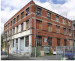
fitzroy argyle street fitzroy argyle street 110
