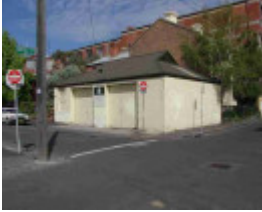
fitzroy argyle street fitzroy argyle street 118-120 unit 3
