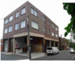
fitzroy chapel street fitzroy chapel street 45-47
