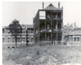
Fairfield Hospital Wards - Exterior
