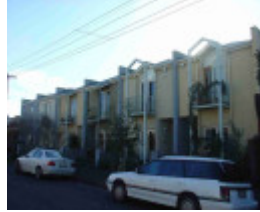
Fitzroy North Woodside Street 9-21.JPG
