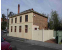
National School - 27 John Street
