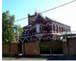
FCJ School Building
