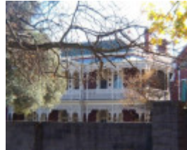
FCJ Convent Building
