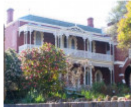
FCJ Convent Building
