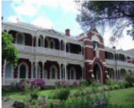
FCJ Convent Building
