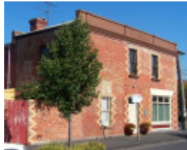
Significant signage on rear and side walls.JPG
