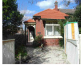
Fitzroy North McKean Street 262 v2.JPG
