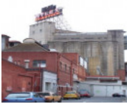
Barrett Burston Richmond Maltings
