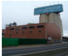
Barrett Burston Richmond Maltings
