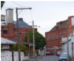
Barrett Burston Richmond Maltings
