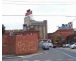
Barrett Burston Richmond Maltings
