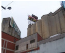
Barrett Burston Richmond Maltings
