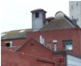
Barrett Burston Richmond Maltings
