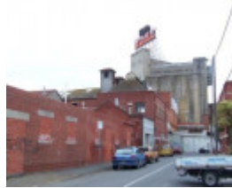
Barrett Burston Richmond Maltings
