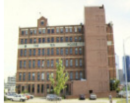
1 robur tea building clarendon street south melbourne rear view dec1992
