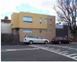
fitzroy north barkly street fitzroy north barkly street 1a
