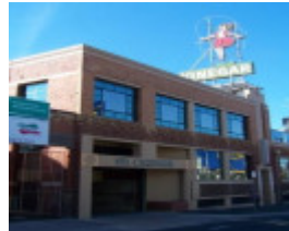
Crusader Plate Building
