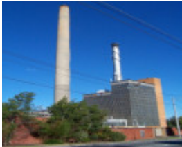
APM Boiler House
