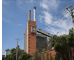
APM Boiler House
