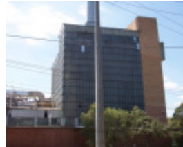
APM Boiler House
