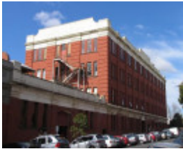
70 Oxford Street - west elevation from Oxford Street
