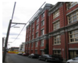
125 Oxford Street - view from Little Oxford Street
