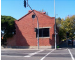
Fitzroy Gas Works Valve House
