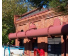
Fitzroy Gas Works Valve House
