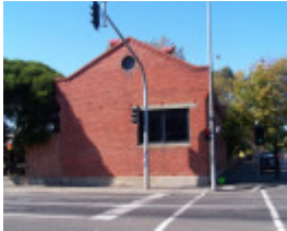
Fitzroy Gas Works Valve House
