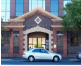
Melbourne Tramway & Omnibus Cable Tram Depot
