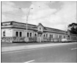
Cable Car Engine House Shed
