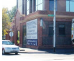
Melbourne Tramway & Omnibus Cable Tram Depot
