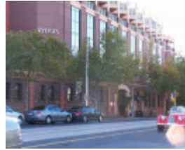
Melbourne Tramway & Omnibus Cable Tram Depot
