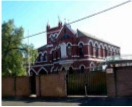
FCJ School Building
