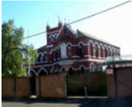
FCJ School Building
