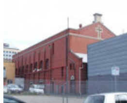
Cathedral Hall view from Young St
