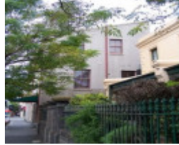
Royal Terrace - 49 Brunswick Street (rear)
