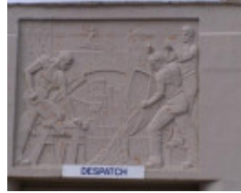
Former Builders Steel Form Supply
