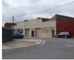
Former Builders Steel Form Supply
