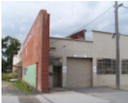
Former Builders Steel Form Supply
