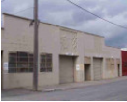
Former Builders Steel Form Supply
