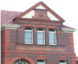
Richmond North Primary School
