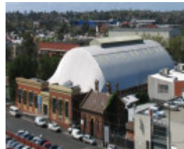
Gas Inspector's Residence and Richmond Baths
