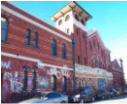
New Australian Electric Lighting Co. Power Station
