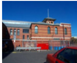
New Australian Electric Lighting Co. Power Station
