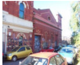
New Australian Electric Lighting Co. Power Station
