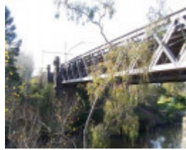
Hawthorn Railway Bridge
