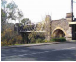
Hawthorn Railway Bridge
