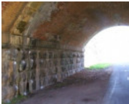
Hawthorn Railway Bridge
