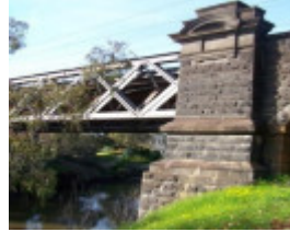
Hawthorn Railway Bridge
