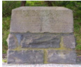
Deep Rock Swimming Club site - foundation stone
