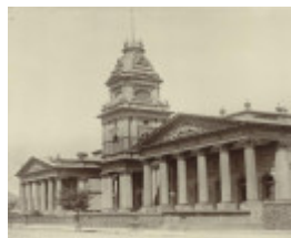
Town Hall Exterior
