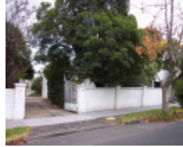
Fairfield Park Crescent 55(1).JPG
