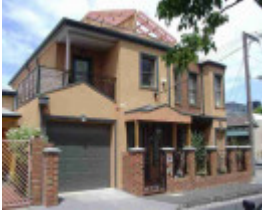
richmond miller street richmond miller street 29
