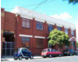
clifton hill groom street clifton hill groom street 37 unit 1-7
