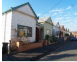
Davis' houses - Mitchell Street
