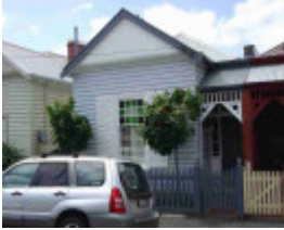
Davis' houses - 5 Mitchell Street
