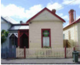
Davis' houses - 7 Mitchell Street
