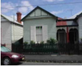
Davis' houses - 8 Mitchell Street
