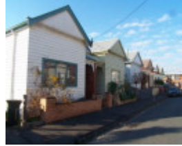
Davis' houses - Mitchell Street
