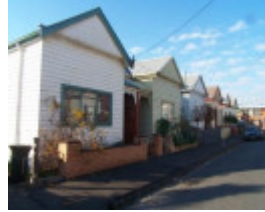
Davis' houses - Mitchell Street
