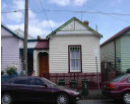
Davis' houses - 10 Mitchell Street
