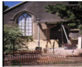
former methodist church ford street beechworth detail front
