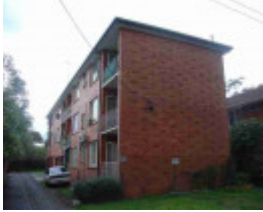
fitzroy north brennand street fitzroy north brennand street 14 unit 1
