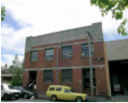
fitzroy north grant street fitzroy north grant street 2-6
