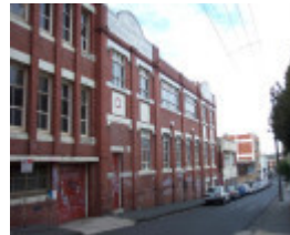
Collingwood Perry St rear 35 johnston St.JPG
